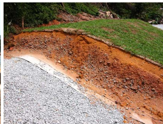
Final Soil Capping System at Base of Landfill
