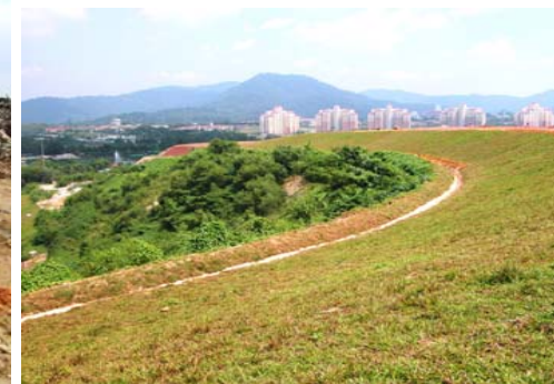
Final Soil Capping System on Side Slopes of Plateau
