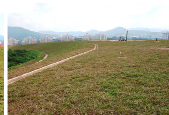
Final Soil Capping System on Side Slopes of Plateau
