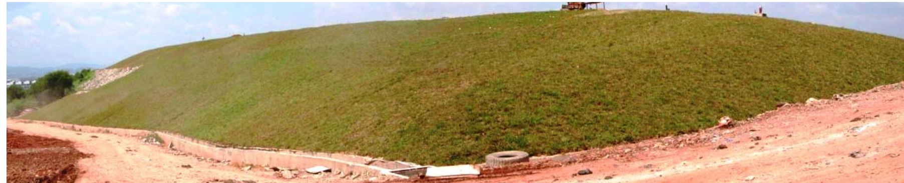
Final Soil Capping System at Plateau of Landfill
