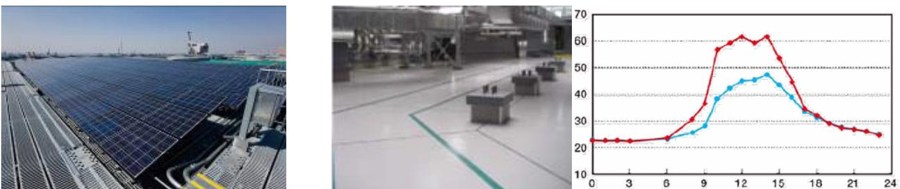
Figure 8. Solar cells and cool roofing (hourly difference of the surface temperature with and without coating)
