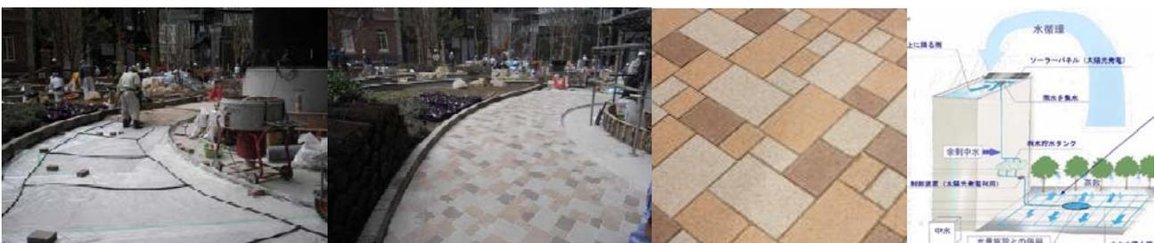
**Figure 11. Moisture-retentive pavement and rainwater recycling system**
