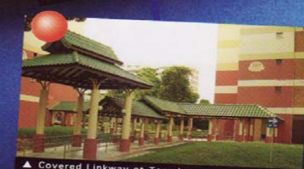
▲ Covered Linkway at Tampines Street 11
