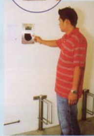
The key to water savings - Residents or contractors will need to flash the stored-value card at the console before they can use the taps.
