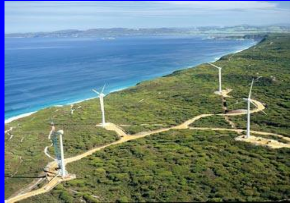
Albany wind farm, Western Australia.
