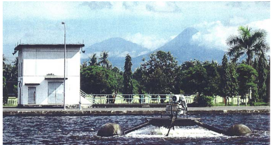
Wastewater treatment plant in Bantul
